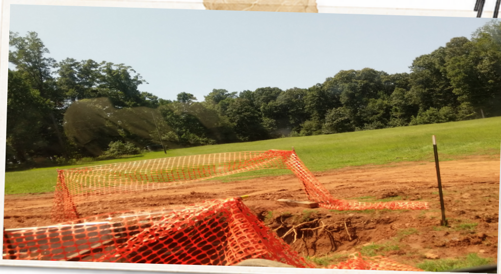
Boundary work in progress. Trench for utilities. A line that will soon become a fence.
