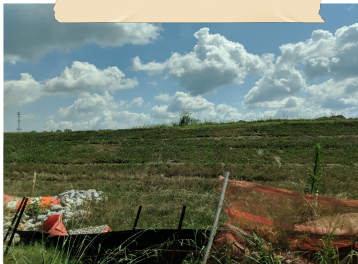
Graded embankment along a future entrance. Somewhere in Barrow County, July 2026.
